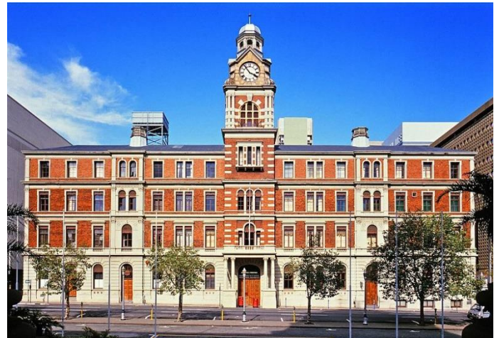
SAPO once occupied this Johannesburg building, which was designated a national monument in 1978. Source: Wikimedia.
